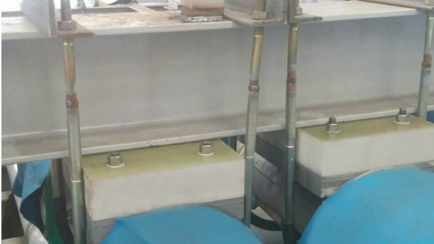
Figure 1. LNG pipe insulated from super structure I-beam with NP500CR.
