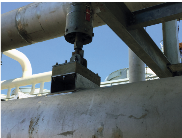
Figure 3. NP500CR insulates an LNG pipe hanging from an adjustable hanger.
